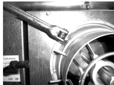
6. Remove air valve from existing VAV unit by breaking the seal around air inlet and the VAV unit. Once it is loose, remove air valve (see Figure 5, p. 13).
